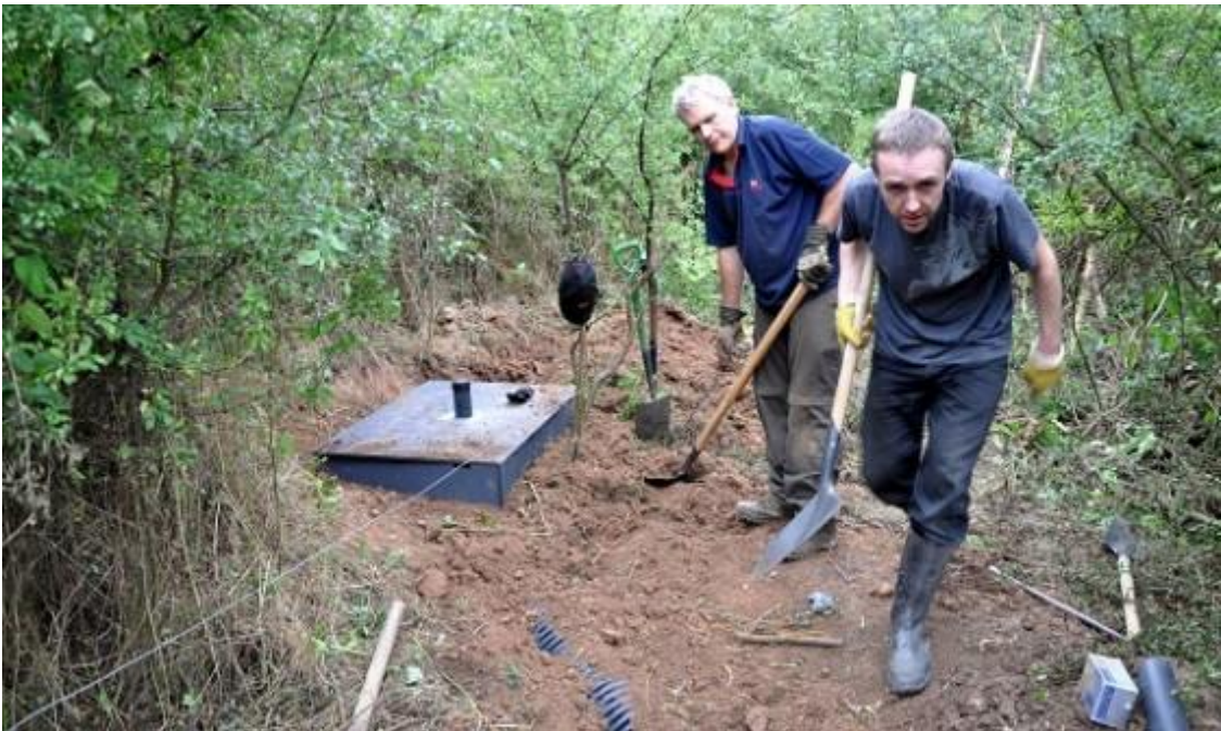
Otter holt installation Upper Catchment (Image: Ruairí Ó Conchúir)
