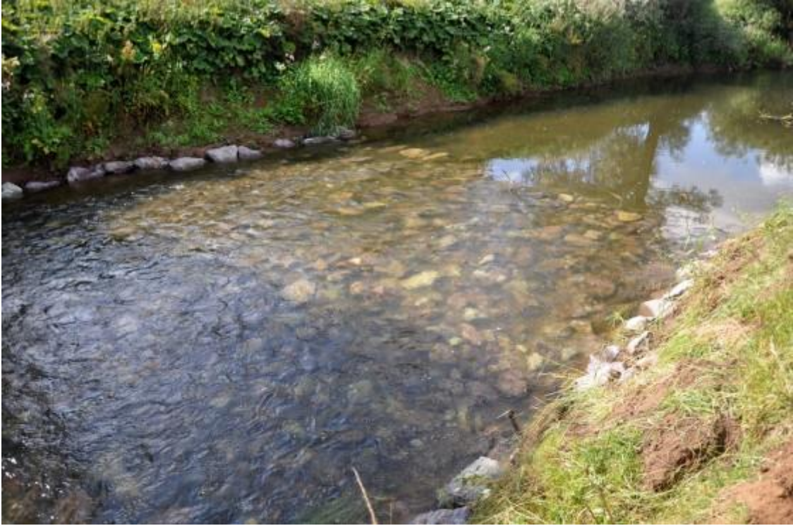
1 of 14 new rubble mats completed on Mulkear in the Summer of 2013 (Image: R. Ó Conchúir)
